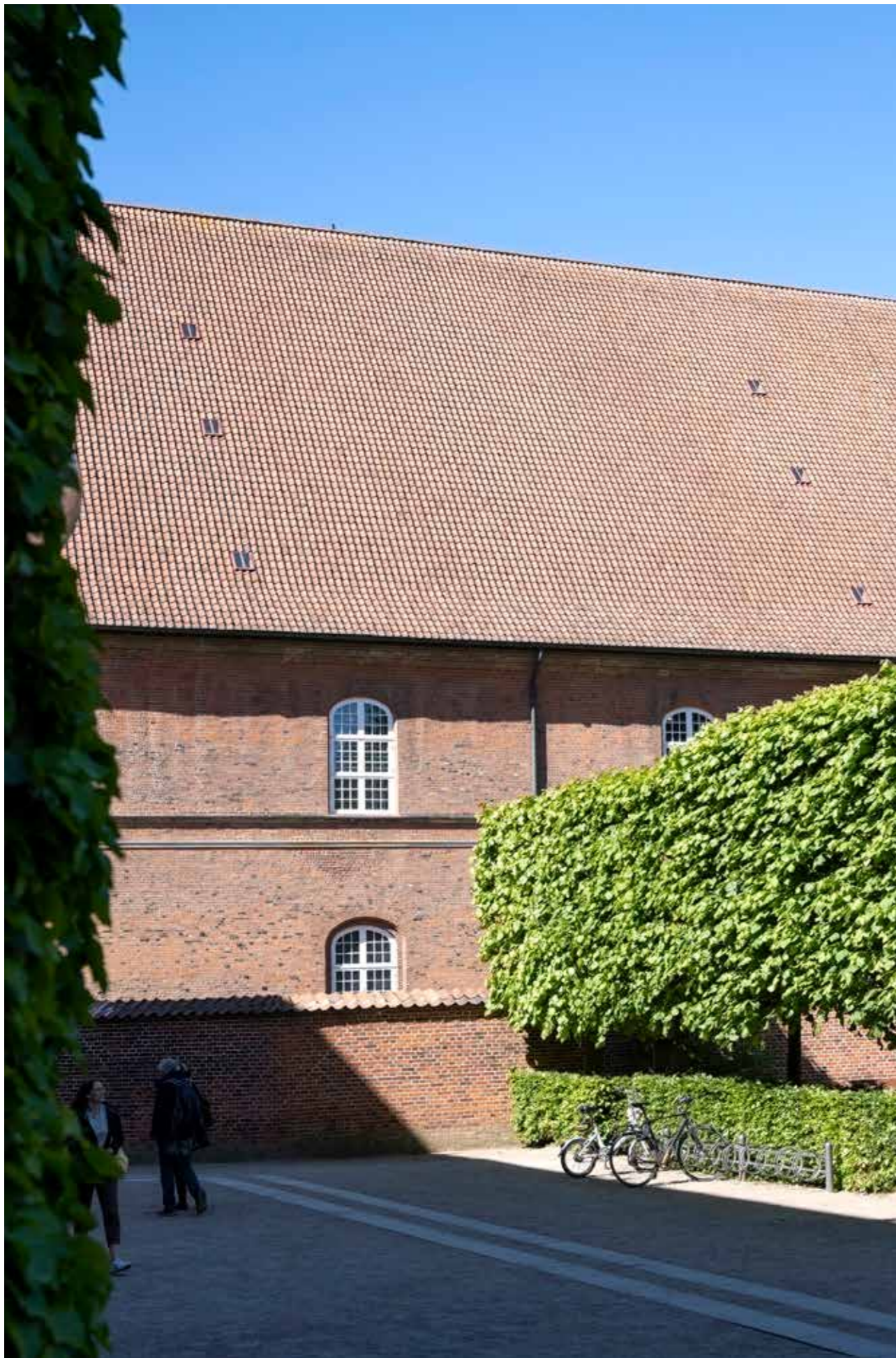
9-tile spacing uninsulated roof windows, Dantegl, Monier hand-curved pantiles at the Christian IV brewery in Copenhagen.
