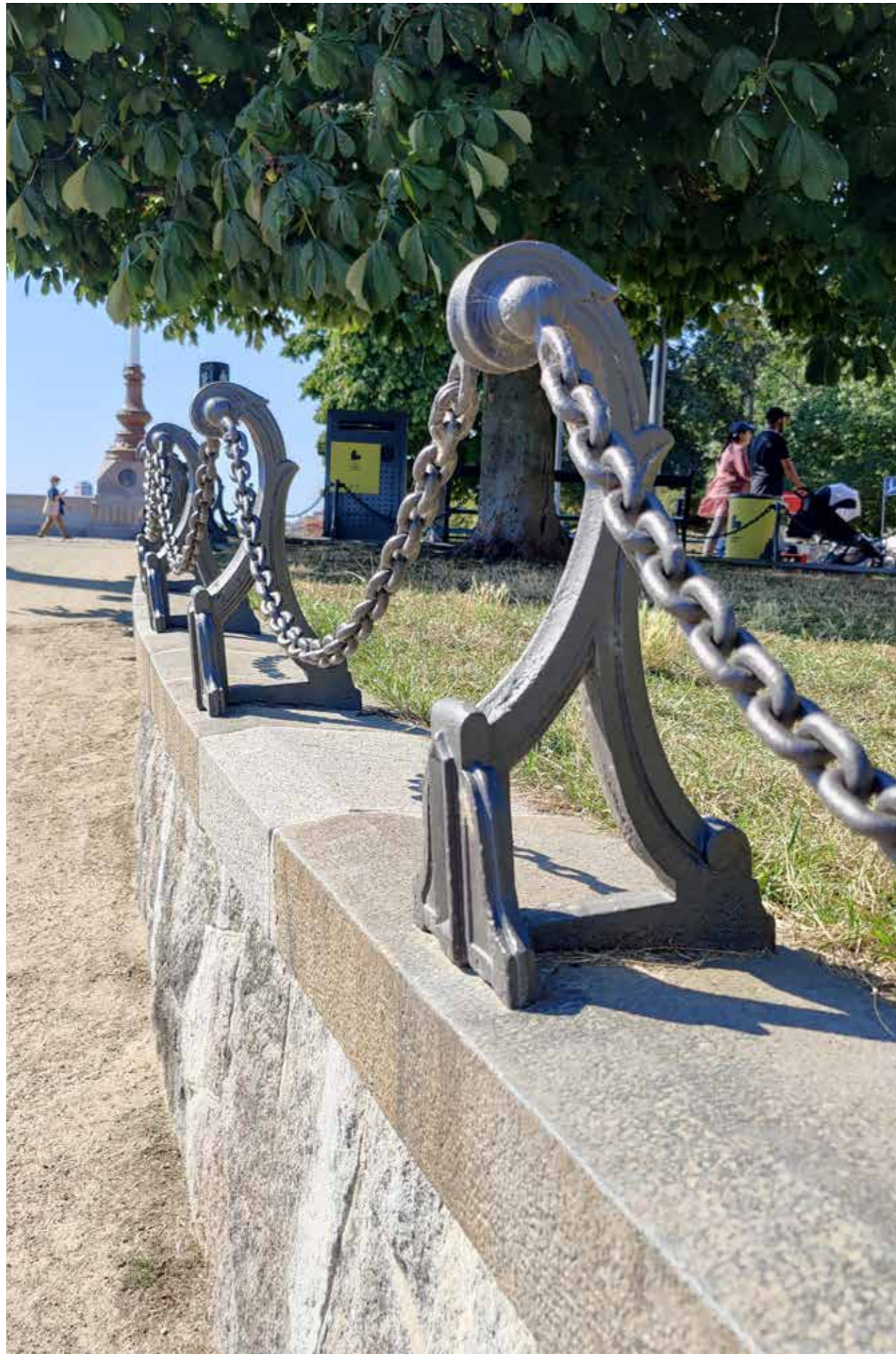
During the renovation of Queen Louise's Bridge, we renovated the goose-necks that are a feature of the handrails along the four paths beside Søerne (the Lakes) in Copenhagen.
