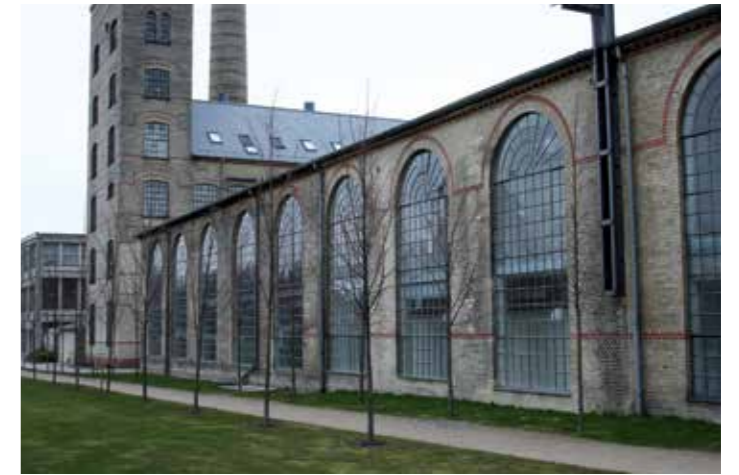
Windows for Brede Værk in Kongens Lyngby north of Copenhagen. The windows are about seven metres tall and also feature a semicircular arch with fanned muntins at the top.
