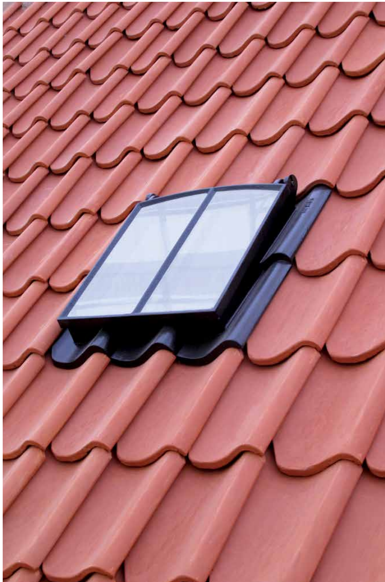
6-tile spacing cast iron roof windows with single vertical muntin, Dantegl, Monier JP2 hand-curved pantiles. Newly laid in 2020 as part of the ongoing renovation of the Nyboder district in Copenhagen.
