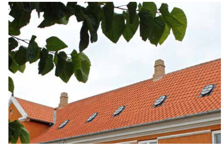
9-tile oval coupled roof windows, Dantegl, Monier pantiles at Prinsens Gård, Frederiksberg Gardens.
