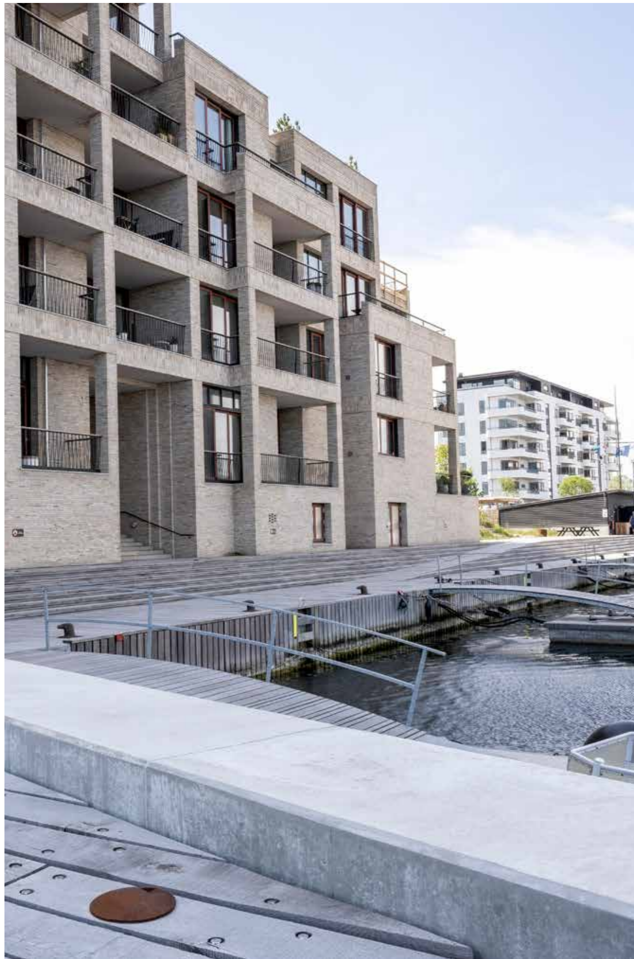
Path Lights along the quay as a feature of the Strandengen project at Copenhagen's Tuborg Harbour.
