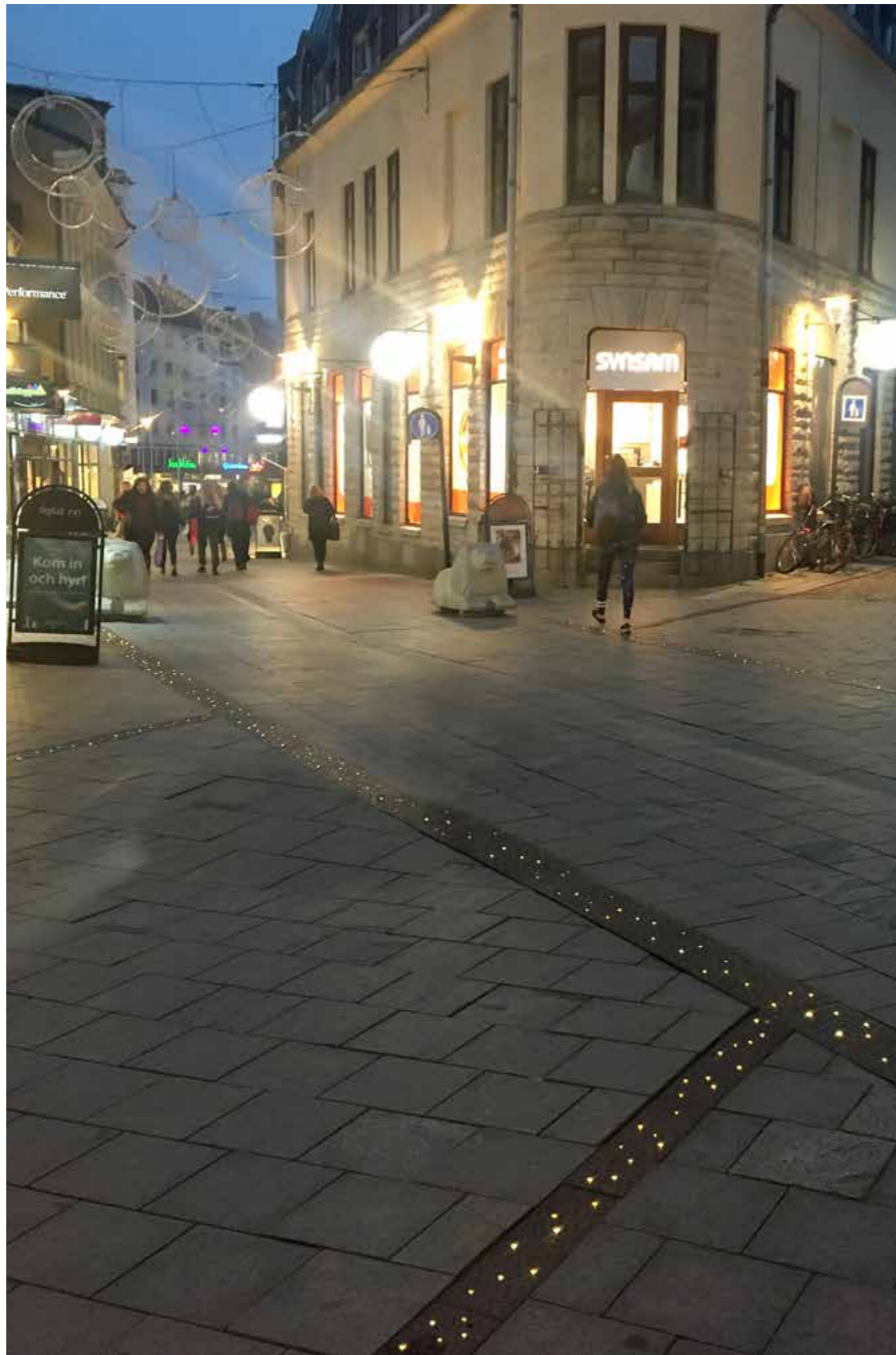
Linköping pedestrian street, Sweden. Campus Lighting Strip is a cast iron paving slab with integrated lighting that is used to indicate special routes or locations in an urban space.
