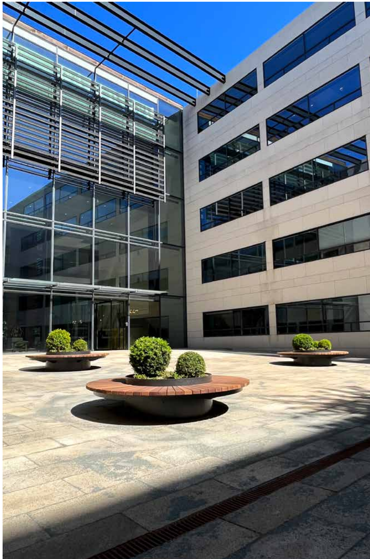
The Platea Round Bench with Planter is installed at Christianshavn in Copenhagen.
