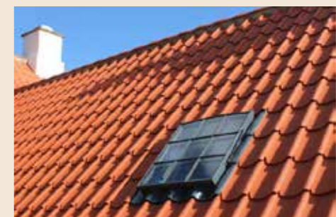
FACADE AND ROOF WINDOWS HISTORICAL CASTINGS
